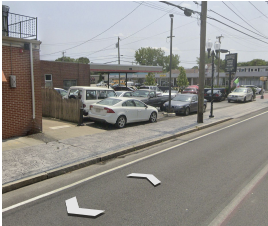
Typical sidewalk condition
